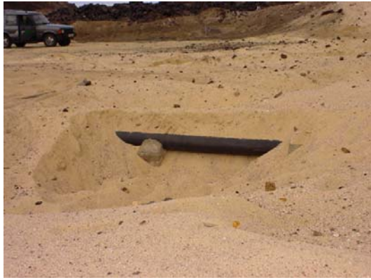
Photo 9: Pipes at Power Station Beach
