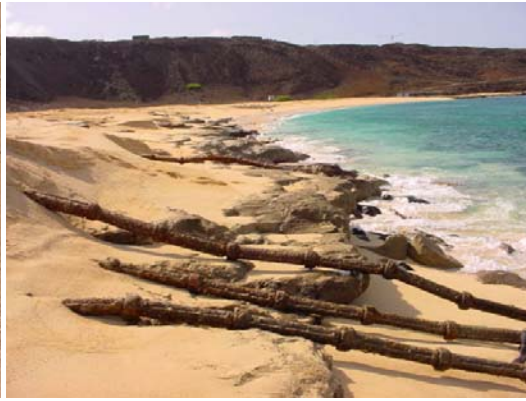
Photo 10: Pipes at Southwest Bay, since removed.
